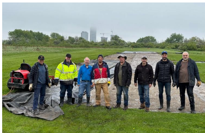
Removal of the old Geo-textile material on a dreary day!
